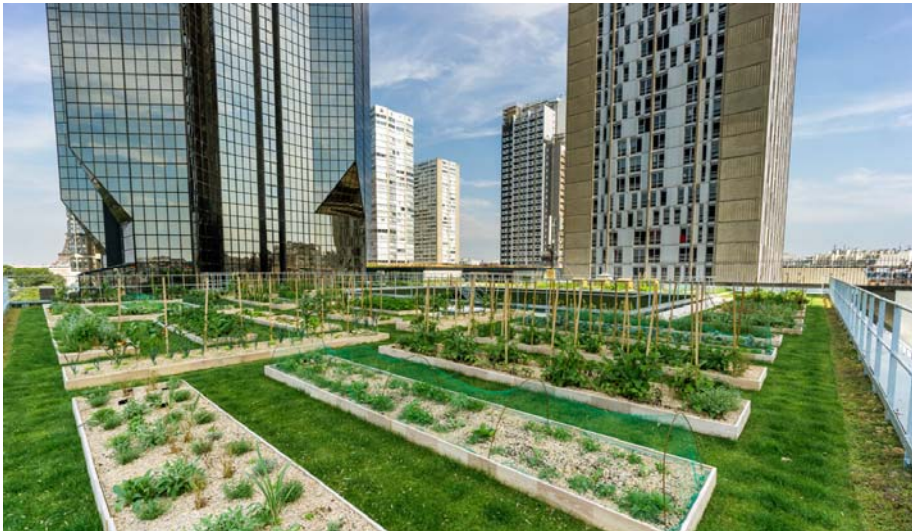
This unique roof garden with a size of roughly 800 m 2 is currently one of the largest in Paris.
