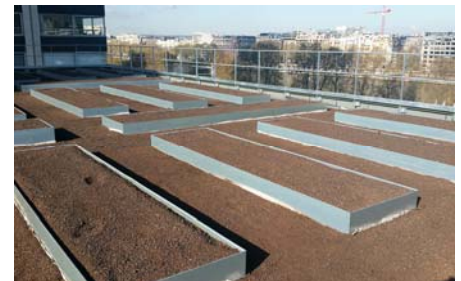
The system substrate "Lawn" was chosen for the entire roof surface.
